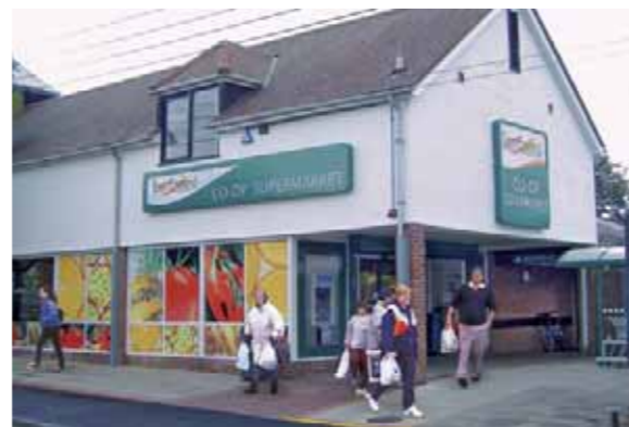
The refurbished West Mersea Supermarket.
